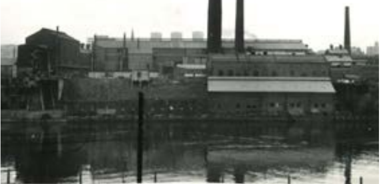
The Leadworks taken from south of the River, October 1965
