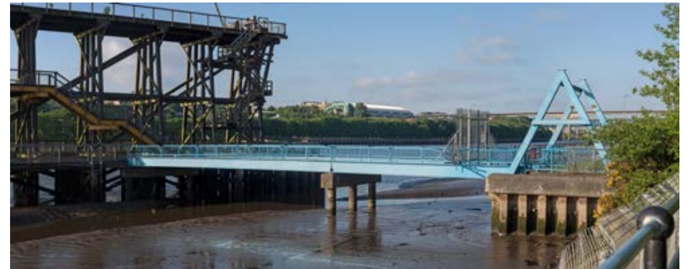
Looking across the river towards Forth Yards from Dunston Staiths (Scheduled Monument and Grade II listed structure).
