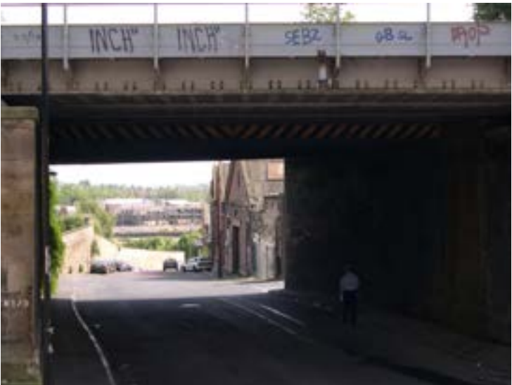
Framed views and shady gateways through legacy Railway infrastructure.
